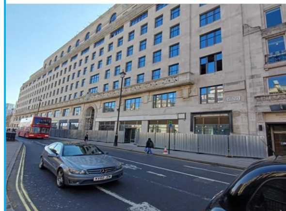
Scaffolding Strike to Street Level
